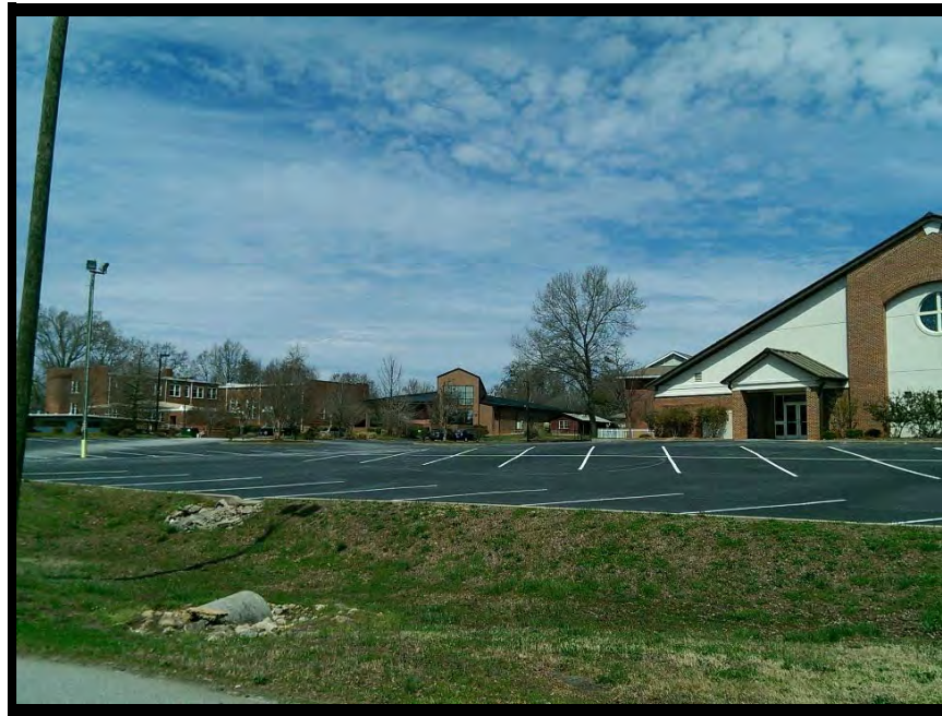
North view from site
